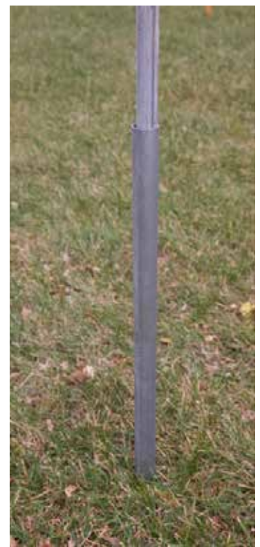
3. A smaller diameter pole can be inserted into a 2.5-ft. anchor pipe.
