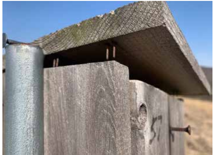
Thin wood roofs that are stapled on can warp and pull up from sides. (Gene Kroupa)
